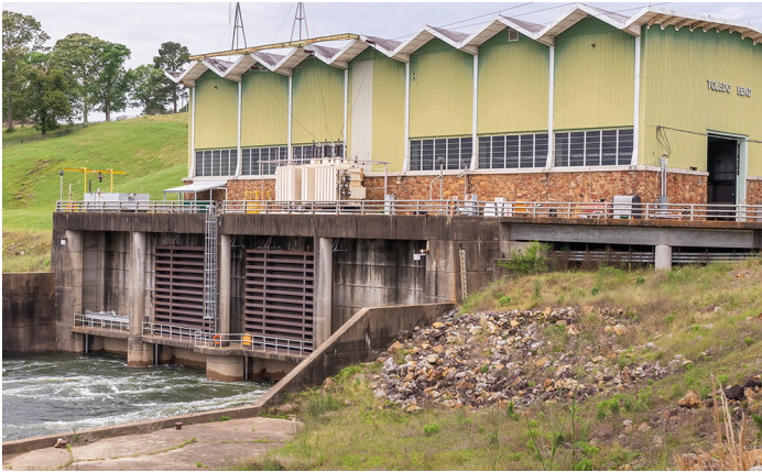
Figure 20. Hydroelectric plant at Texas end of Toledo Bend Dam (Heart of Louisiana) 43 .
